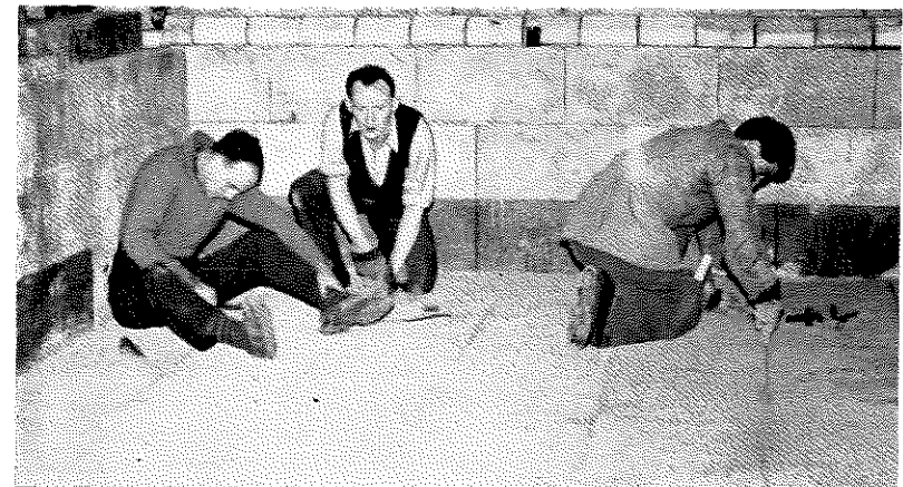
● Messrs. Urwin, Kelly and Bailey of Glasgow Works on the final stages of compacting the bottom of No. 50 F.
